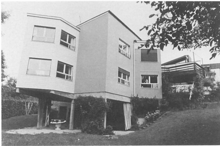
7. Schmitz house, Biberach, 1950, one of a pair which were Häring's last executed works. The space between the concrete legs was originally left open, allowing a more dynamic connection with the garden.
