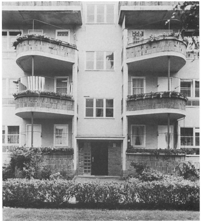
4. Housing at Siemensstadt, Berlin, notable for its colourful expressed construction in contrast with the smooth white render found elsewhere in the development. Häring's slab blocks run north-south perpendicular to the street, with gardens between.
